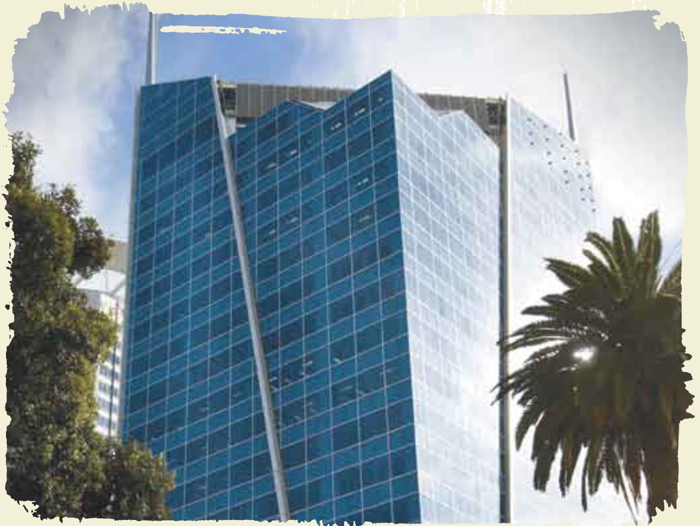
Lumley General New Zealand's new environmentally-friendly building in Auckland.
