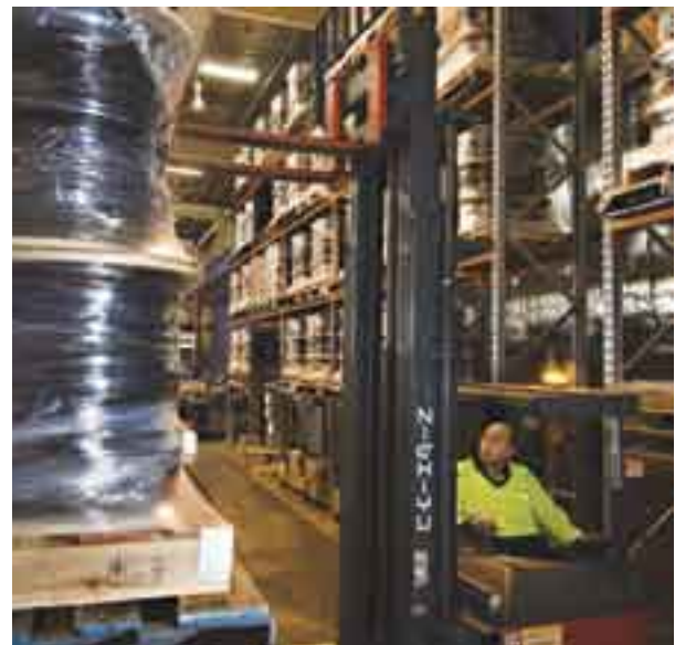
New pallet racking at Bakers Construction and Industrial, Blacktown.
