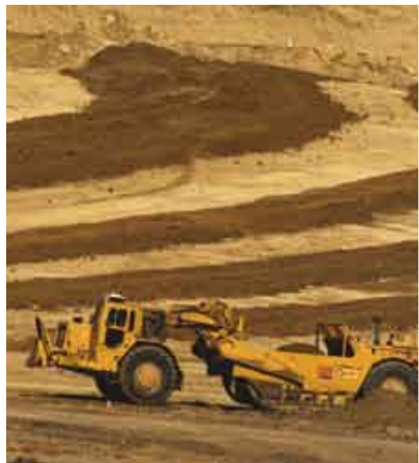
Rehabilitation in progress at Curragh.
