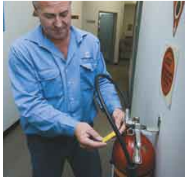
Health and Safety Representative Ashley Bush conducting a workplace inspection.
