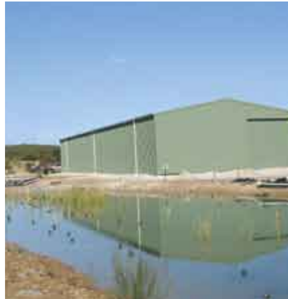
New hatchery building at the research aquafarm adjacent to the mine.
