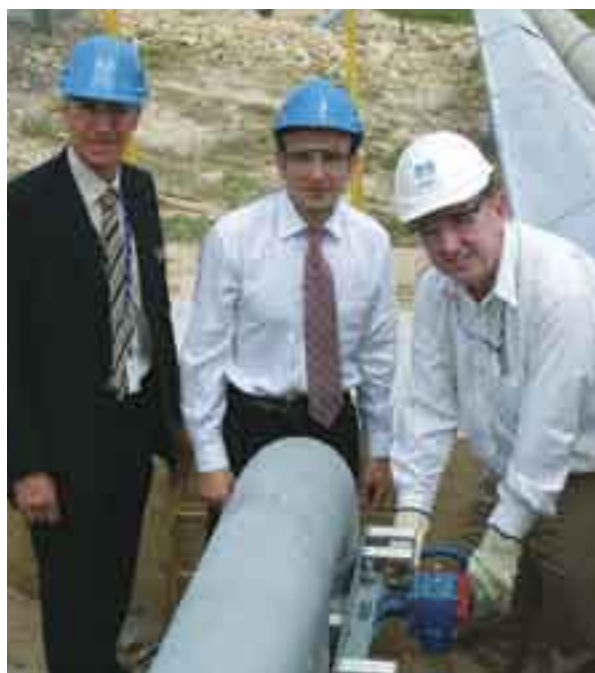
CSBP Managing Director, Keith Gordon, is joined by Max Viscovich (left) and Ross Mignacca (centre) from the WA Water Corporation at the Kwinana Water Reclamation Plant valve-turning ceremony.
