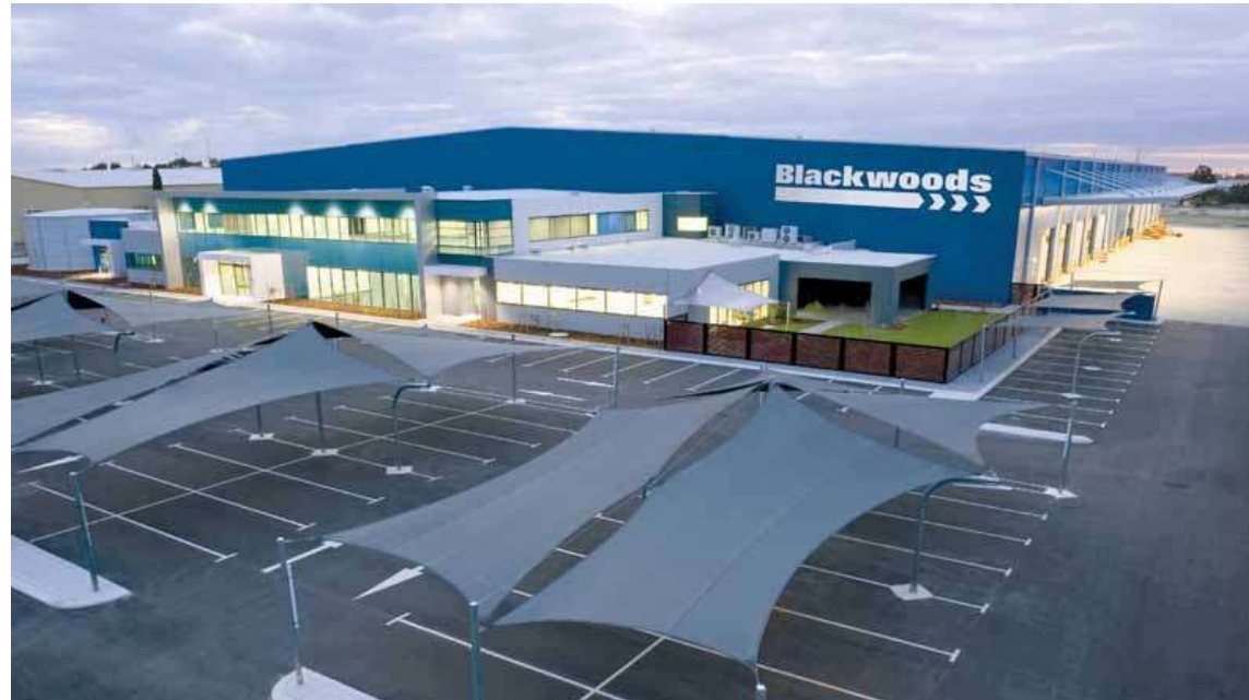
Blackwoods Perth Distribution Centre
