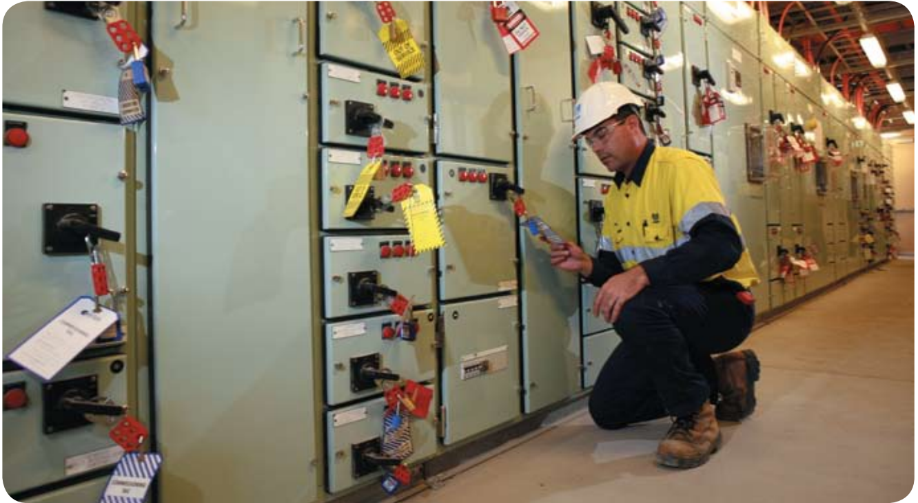
▲ CSBP Process Technician Mike Perry inspects isolation locks which were introduced to our permit to work system this year.
