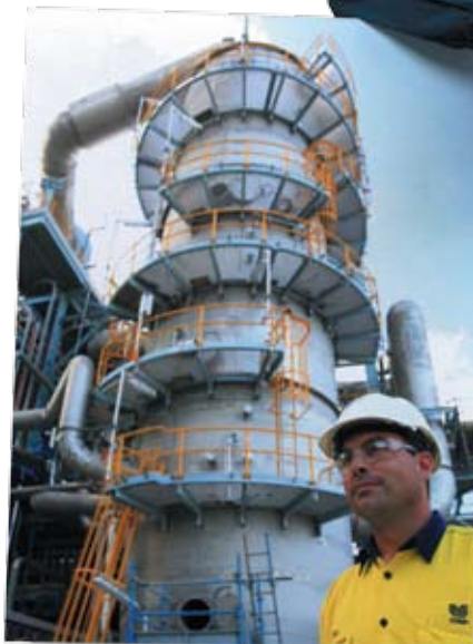
CSBP Process Technician Mike Perry at the new Kwinana ammonium nitrate facility.
